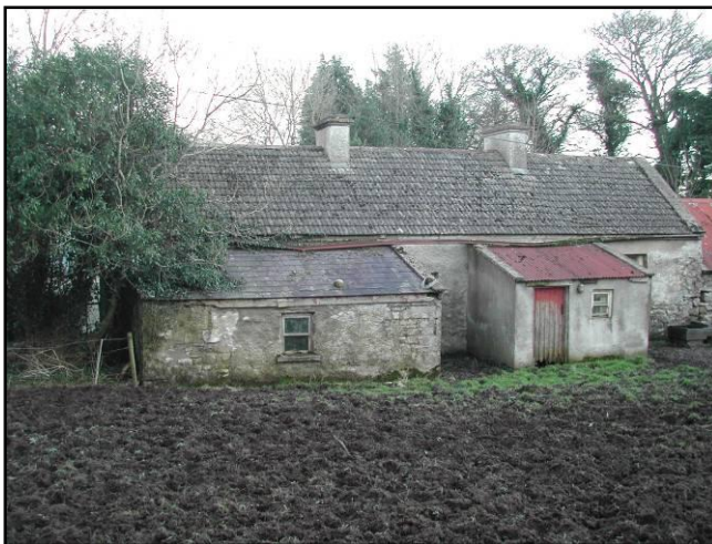
Plate 8 The farmhouses to the north of Aghalenane/Ardloy Loughs would be lost as a result of the proposed development. These are used as a roost for Soprano pipstrelles.
